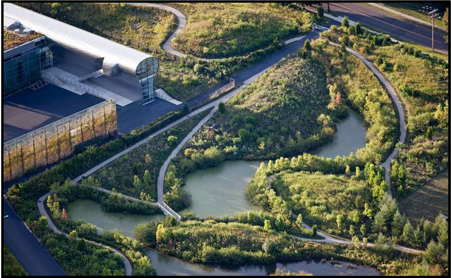
Whitney Water Purification Facility, New Haven, Connecticut, USA .
